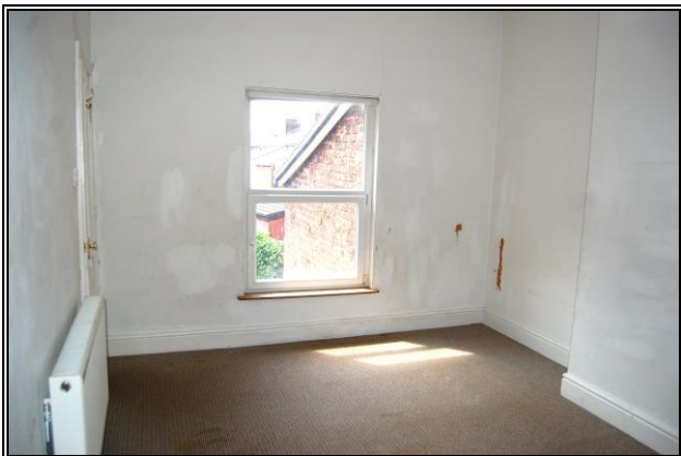
First Floor Flat Bedroom
